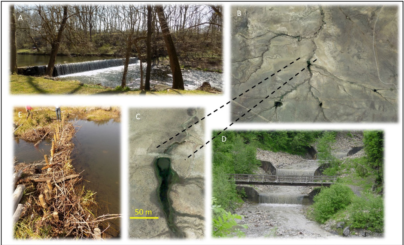
FIGURE 2 | Examples of types of human dams discussed here. (A) A mill dam in Pennsylvania, USA. (B) A river network with multiple earthen embankments in semiarid southern Wyoming, USA. (C) A close-up of one of these embankments. (D) Check dams in the Alptal region of Switzerland. (E) A beaver dam analogue in South Park, Colorado, USA.
