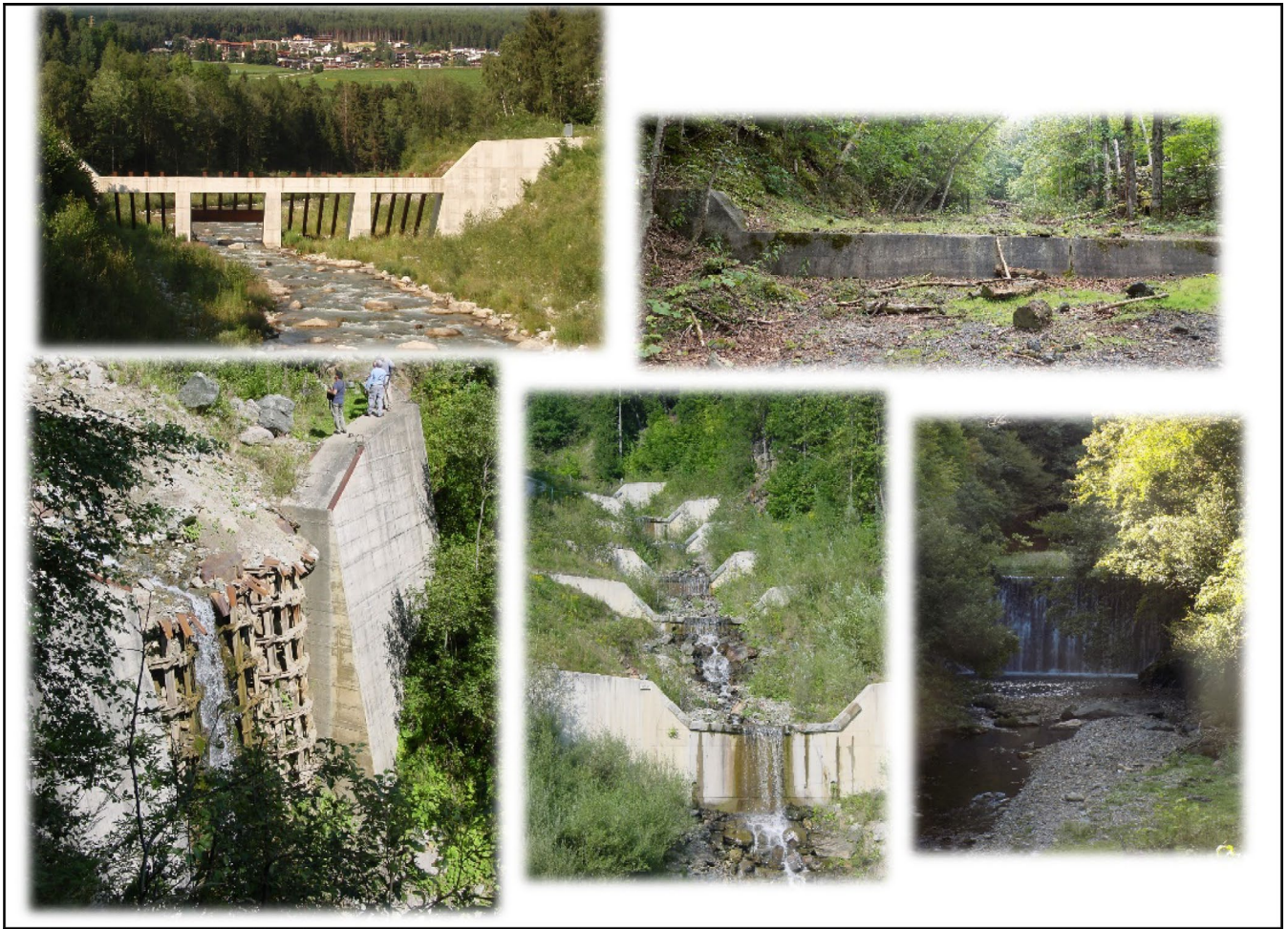
FIGURE 5 | Examples of different types of check dams. Upper left, open check dam in Italy; lower left, open check dam (although filled with sediment) in Austria. Upper and lower right, low (~1 m tall) and high (~6 m tall) closed check dams, respectively, in Japan. Lower center, a sequence of closed check dams in Austria.
